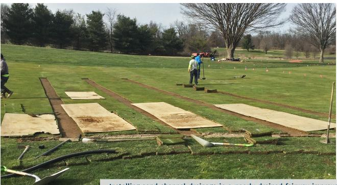
Installing sand channel drainage in a poorly drained fairway improved playing conditions and turf health and greatly reduced cart restrictions.
