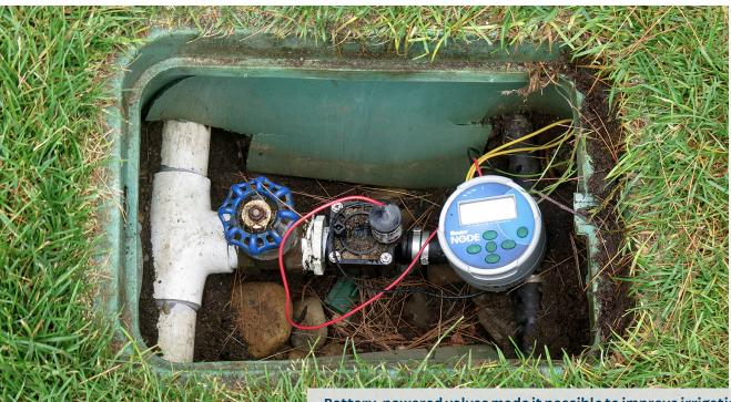
Battery-powered valves made it possible to improve irrigation coverage and control in green surrounds at minimal cost.
