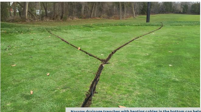
Narrow drainage trenches with heating cables in the bottom can help prevent winter injury on putting greens with poor surface drainage.
