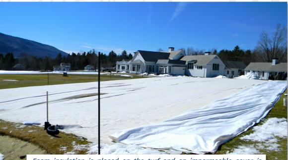
Foam insulation is placed on the turf and an impermeable cover is placed over the foam. Air tubes below the covers provide ventilation.
