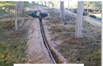
Two loops of in-line drip tubing were installed around the base of each tree on nine holes at Shadow Creek.
