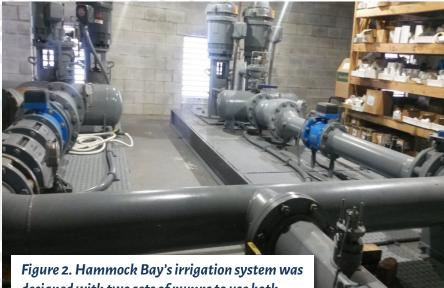
Figure 2. Hammock Bay's irrigation system was designed with two sets of pumps to use both treated wastewater and salty brackish water.
