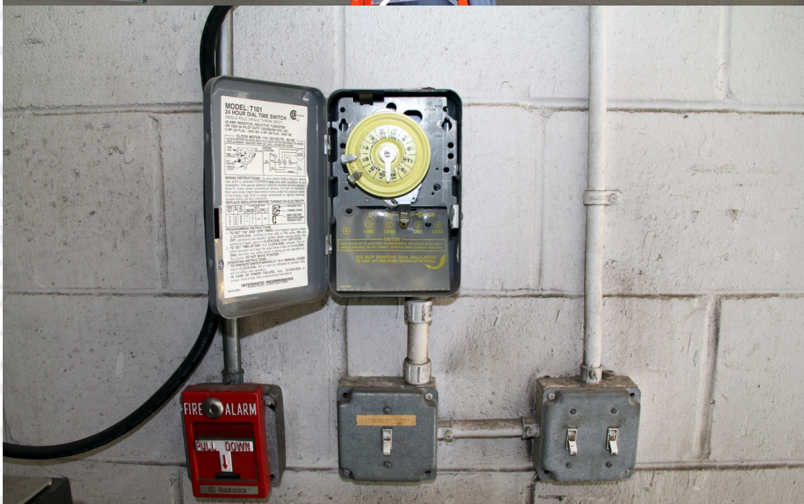
Figure 1. Collectively, small improvements like replacing high-energy-use bulbs with LED lights and installing timers to decrease power use during nonoperational hours can make a big dent in monthly power usage.
