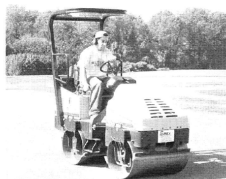
Figure 2. A roller (2970 lbs) was used to create compaction in the test plots.
