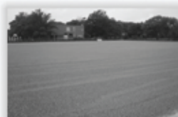
Completed Base for Artificial Field, Baileys Elementary School
