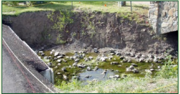
Bank erosion left uncontrolled threatens bridges, roads and impacts water quality.
