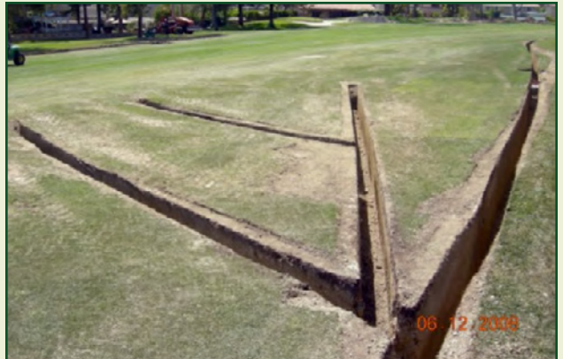
Subsurface drains provide excellent stormwater drainage.
