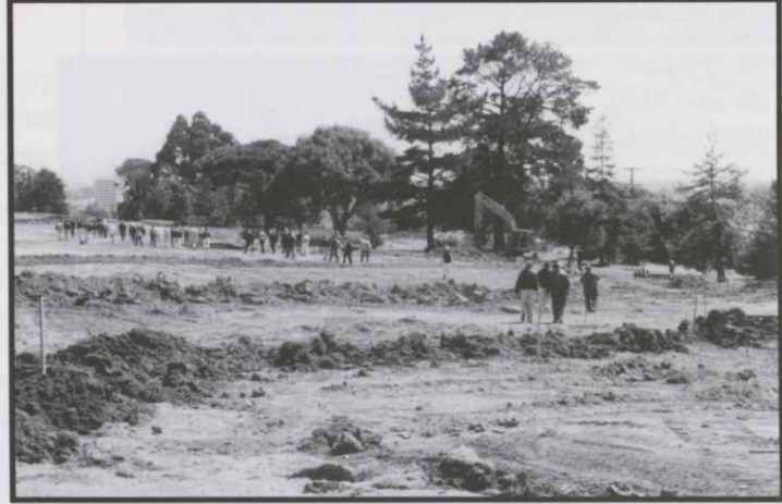
Attendees viewed irrigation and drainage installation work
