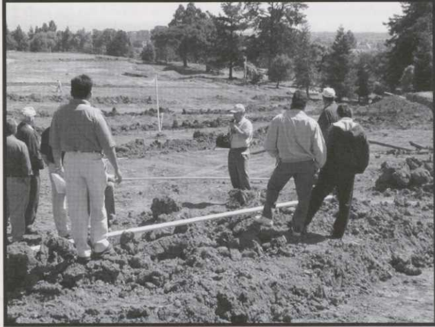
Project Manager Cliff Bechtal describes the drainage work
