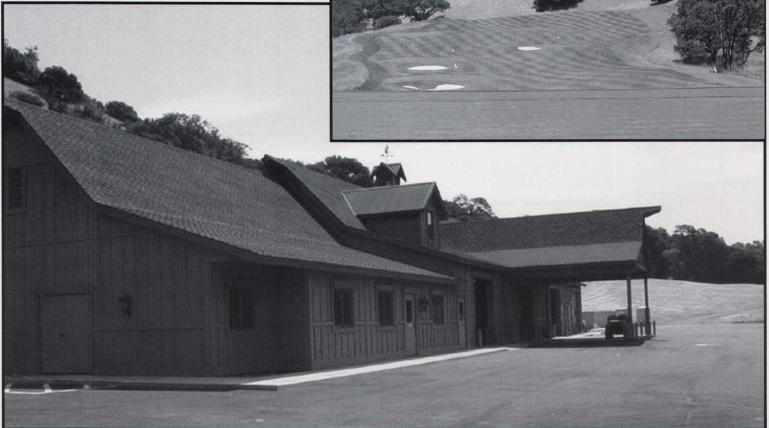
Mayacama's new maintenance facility
