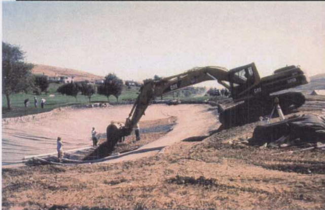
New Lake Construction
