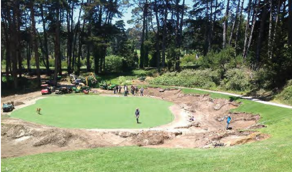
During (above and right): We created bunkers that followed the land's natural contours. GCSANC member Kaminski Golf handled rough shaping.
