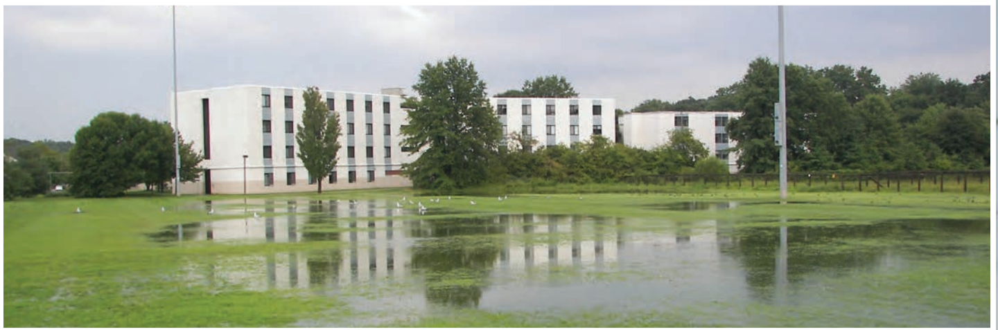
Fields constructed with fine textured soils and built without adequate surface pitch are highly prone to exhibit poor drainage following rain events (Photos by Brad Park).
