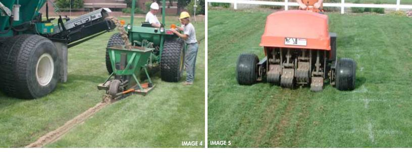
The concept behind the built-up sandcapped system is to combine the advantages of the sand cap system (drainage and sand root zone playing surface) while providing almost uninterrupted availability. The idea is to cut drains in the existing field running lengthwise, put drain tile in the lines, and back fill with pea stone and then sand, or coarse sand alone (Image 3, pg. 13 and Image 4 pictured above).
