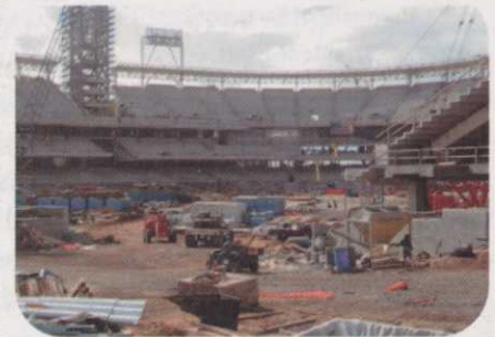
Petco Park - under construction
