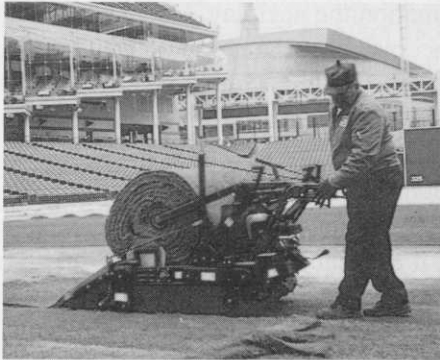
INSTALLED CLEVELAND INDIANS IN 42" AND 48" ROLLS
