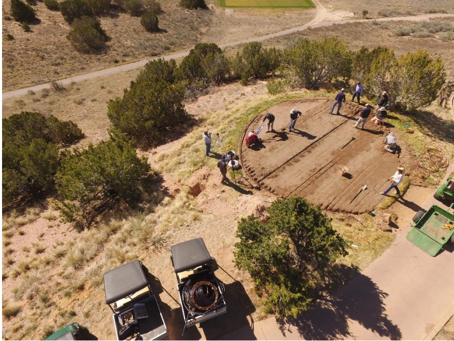
Figure 3. Process of installation with the existing turfgrass removed.
