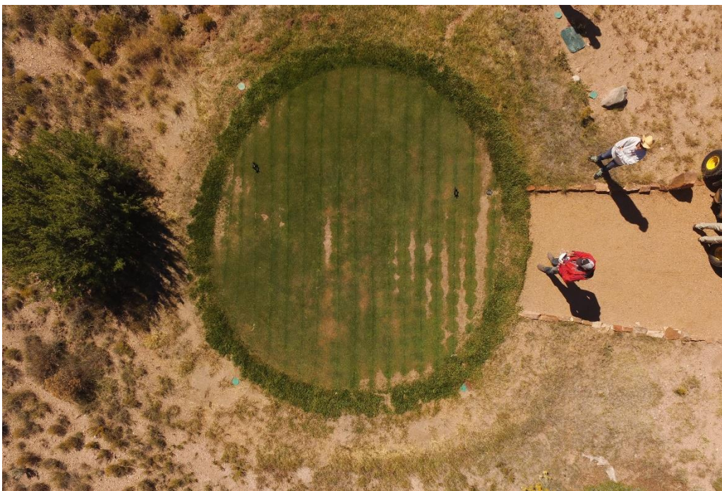
Figure 6. Incorrectly installed subsurface drip irrigation.
