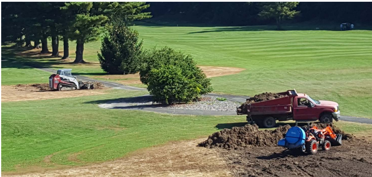
Figure 7. All equipment used in the turf removal and disposal process. Light brown areas have been treated with glyphosate, but not yet “Harley Raked.” Mini-excavator and “Harley Rake” used to remove turf (upper left corner). Dump truck and front-end loader used to transport removed turf to final destination.
