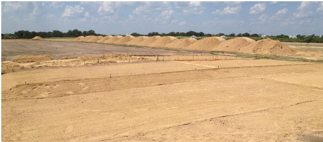
Figure 6. Construction of sand-capping treatments during summer of 2014.
