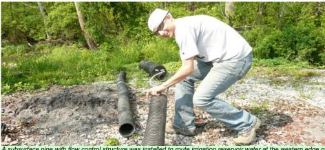
A subsurface pipe with flow control structure was installed to route irrigation reservoir water at the western edge of the course through two corrugated black tiles.
