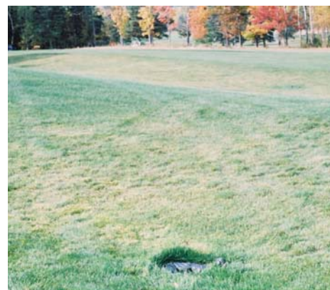
A surface inlet is placed at the bottom of the pothole to rapidly remove water that collects in the depression.
