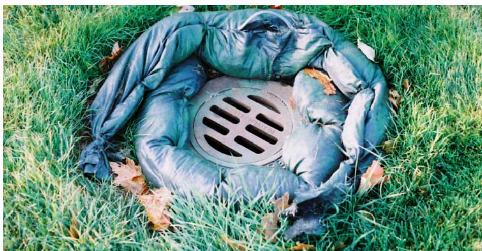
In March of 2011, filter socks were installed around each inlet within the eastern portion of the golf course study area. The filter socks were filled with 75% steel slag, 2.5% cement kiln dust (CKD), and 22.5% silica sand.
