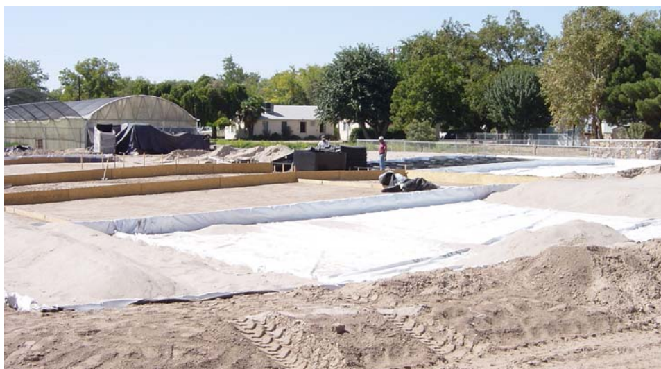
PVC liners were placed between plots to prevent lateral movement of water between plots.
