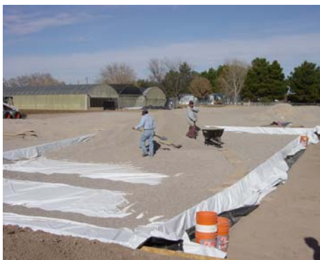
Irrigation research plots were built to study the impact of irrigation type (sprinkler vs. subsurface drip irrigation vs. subirrigation) and type of rootzone mix (straight sand vs. sand mixed with peat vs. sand mixed with urea-formaldehyde polymer) on irrigation efficiency and turfgrass performance of 'Bengal' creeping bentgrass.
