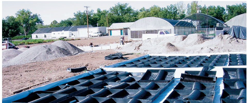
Studies at New Mexico State University are testing the feasibility of subsurface irrigation for putting greens.
