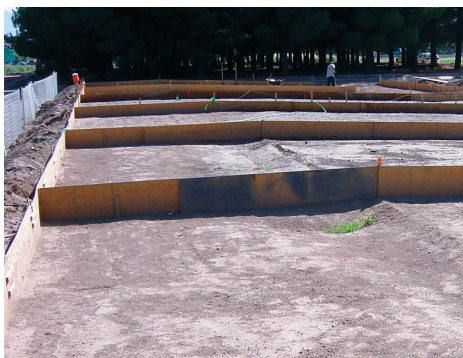
Construction of the subgrade of experimental putting greens at the Fabian Garcia Research Center at NMSU.
