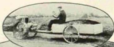
At Left: Centaur with dump cart for haulage.
