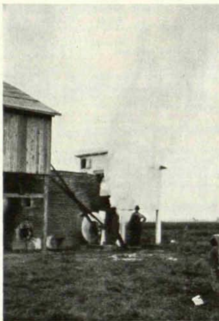
FAN FOR REMOVAL OF VAPORS FROM DRYING DRUM
