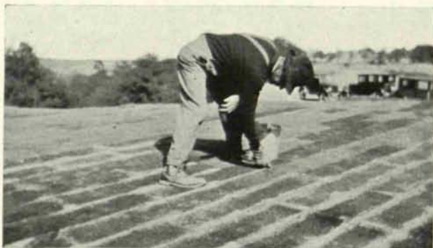
FILLING THE CRACKS WITH COMPOST
