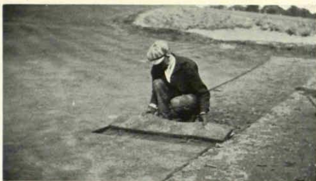
LIFTING SOD ONTO STEEL PLATE TO CARRY TO TRIMMERS
