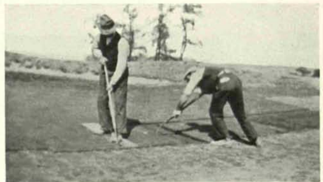
CUTTING AND LIFTING THE SOD
