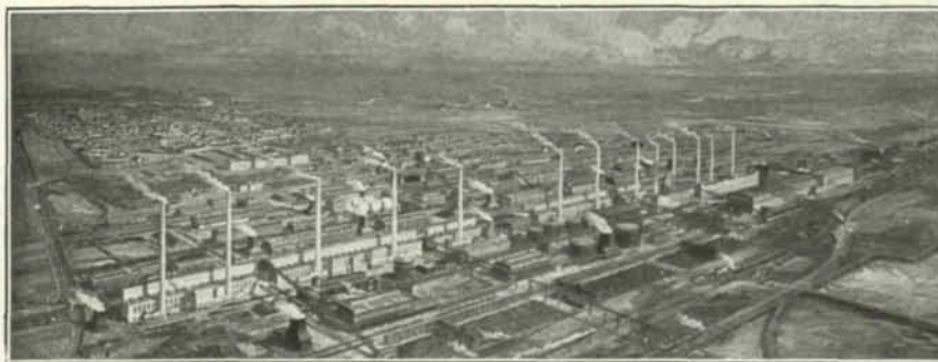
FACTORY OF THE SYNTHETIC NITROGEN PRODUCTS CORPORATION, NEW YORK This is said to be the largest nitrogen factory in the world and covers an area of 1470 acres.
