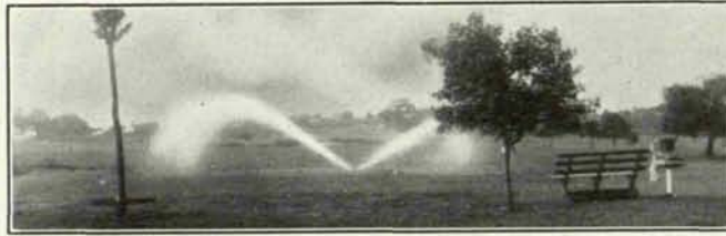
A single installation of a "pop-up" type of rotating sprinkler used to irrigate a tee
