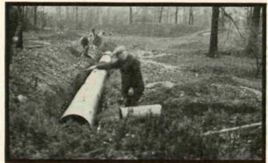
Bert Sheldon, greenkeeper at the Cleveland Country Club, superintending installation of Armco Perforated Pipe on his course
