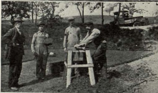
THE CREW AT CHARTIERS HEIGHTS Joseph Ball is the greenkeeper of this Crafton, Pa., course and is very proud of the men who work for him. Lower photo shows Ball on the left supervising the cutting of nursery stock
