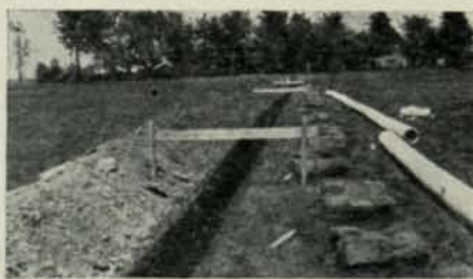
Armco pipe line being laid at the Verity Golf Course, Middletown, Ohio.
