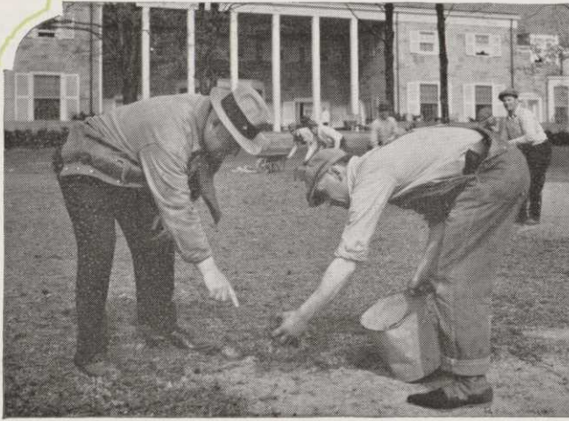
SCATTERING STOLONS. Note the workman in stocking feet to avoid disturbing the seed bed. One live joint should be placed on each square inch of surface.
