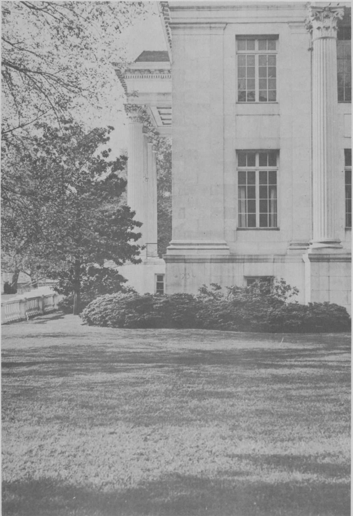
North Lawn. American Red Cross Building. Washington.
