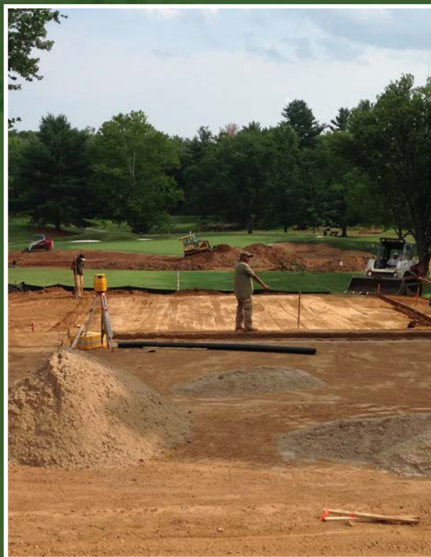
Above: Hole 14 During Construction
