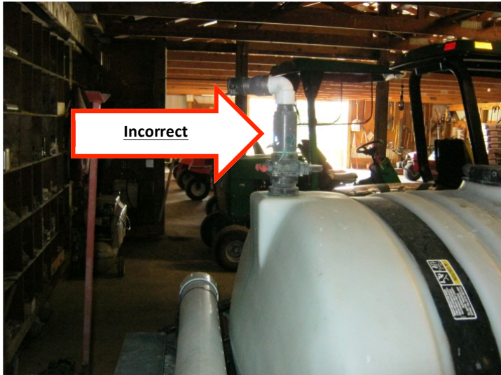
No physical separation in air gap
