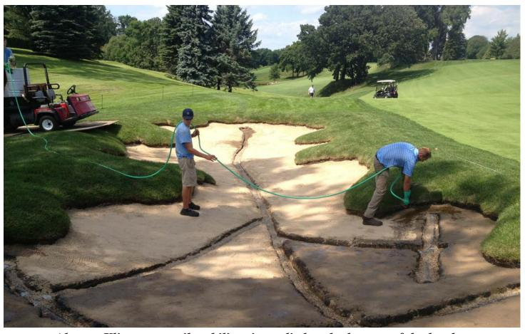
Above: Klingstone soil stabilizer is applied to the bottom of the bunker
