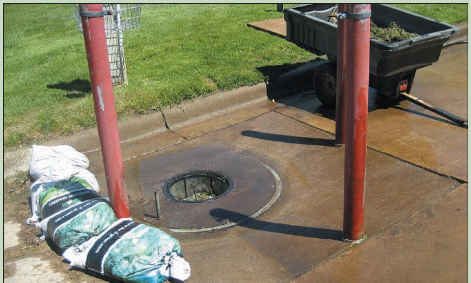
The pictures above show Bob' McKinney's simple wash pad system. He started by sinking a 200 gallon basin into his desired location making sure the area around had sufficient slope. To catch the clippings, a custom made top was put on the basin which would hold a standard screen used for melting products into a sprayer. The rinsate is then discharged on to the turf.
