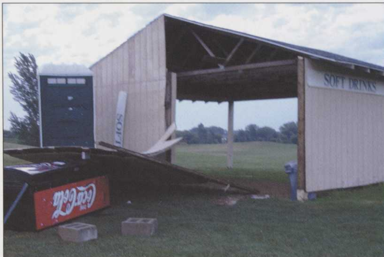
Shelter damage at Heritage Links Golf Club - Paul Eckholm, CGCS
