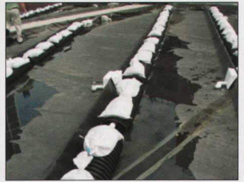
3. Layout of ECS Chambers.
