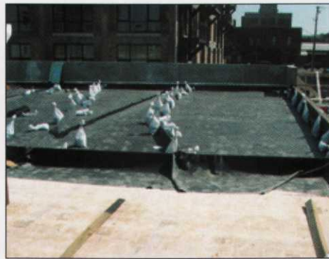
2. ECS Membrane for green roof.
