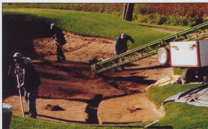
Using the conveyor to empty the bunker.
