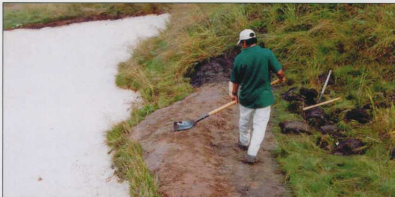
Creating a berm above the bunker to divert water.
