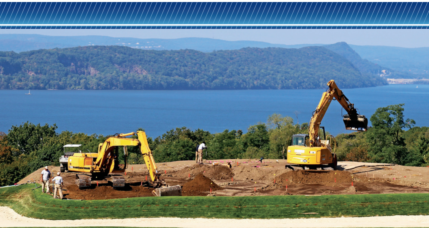
The USGA took 18 months updating the Recommendations for a Method of Putting Green Construction. The recommendations include updates in several areas, including drainage and gravel layer construction.
