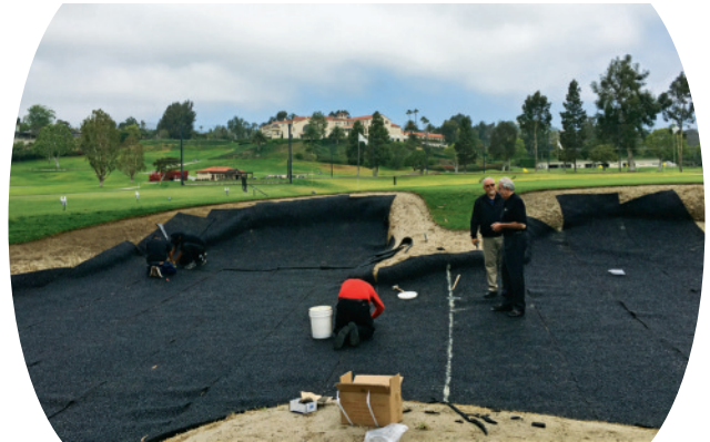
A Polylast bunker liner installation on the practice chipping green bunker at The Riviera CC.
