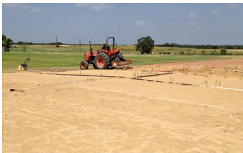
Research plots showing the installation of the sand cap prior to sprigging.
