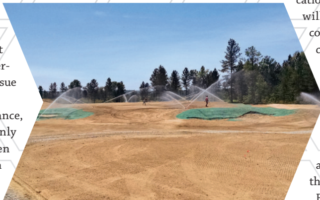
The irrigation design firm Michael Kuhn & Associates, Inc., was hired to help minimize irrigation costs on The Loop's wide fairways. The two-row system installed is designed to keep the water on the maintained turf.
