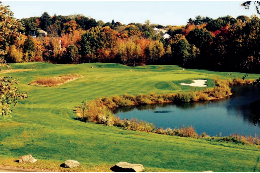
The land for Button Hole, Providence, R.I., was reclaimed from an old junkyard.
