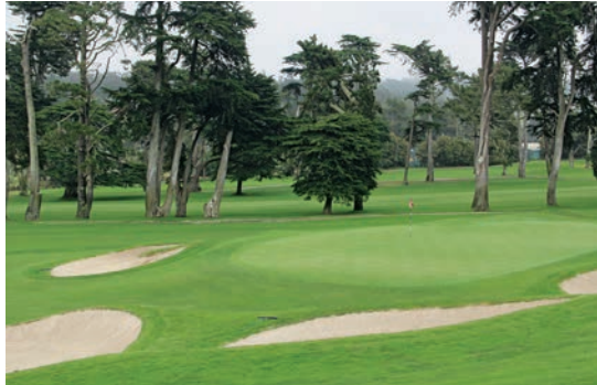
The Olympic Club is installing Capillary Concrete bunker liners in preparation for the 2021 Women's U.S. Open.
