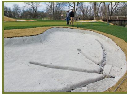
For the bunker renovations Bohn decided to go with Bunker Solutions, a system that uses an artificial turf liner. Plans are to switch all of the bunkers at Wolf Creek to the system.
