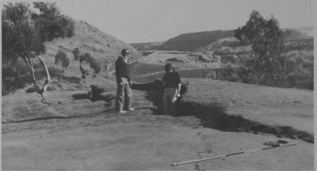
Jim Mercer (above and below left), superintendent at Estrella CC in San Clemente, and Dave Hueber examine part of a 1,000-foot-long crevice opened up on the golf course by a massive land shift.
